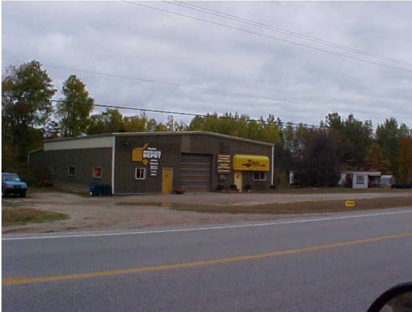
Scheck Signs on M-113, near Clark Rd.
